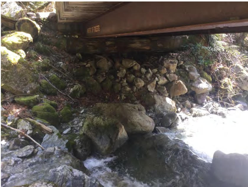
Left Bank Abutment when facing downstream
