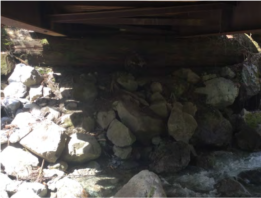
Right Bank Abutment when facing downstream
