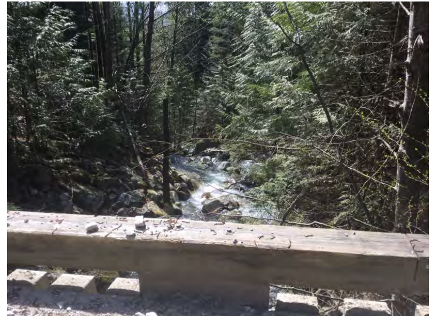
Looking downstream from deck
